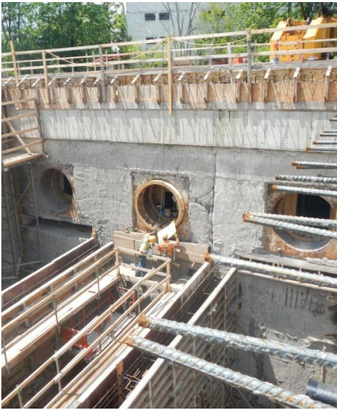
Clinton CSO Storage Facility – Construction June 2013
