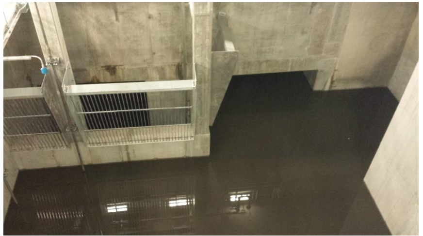
Clinton CSO Storage Facility – Tunnel 1 filling, March 2014
