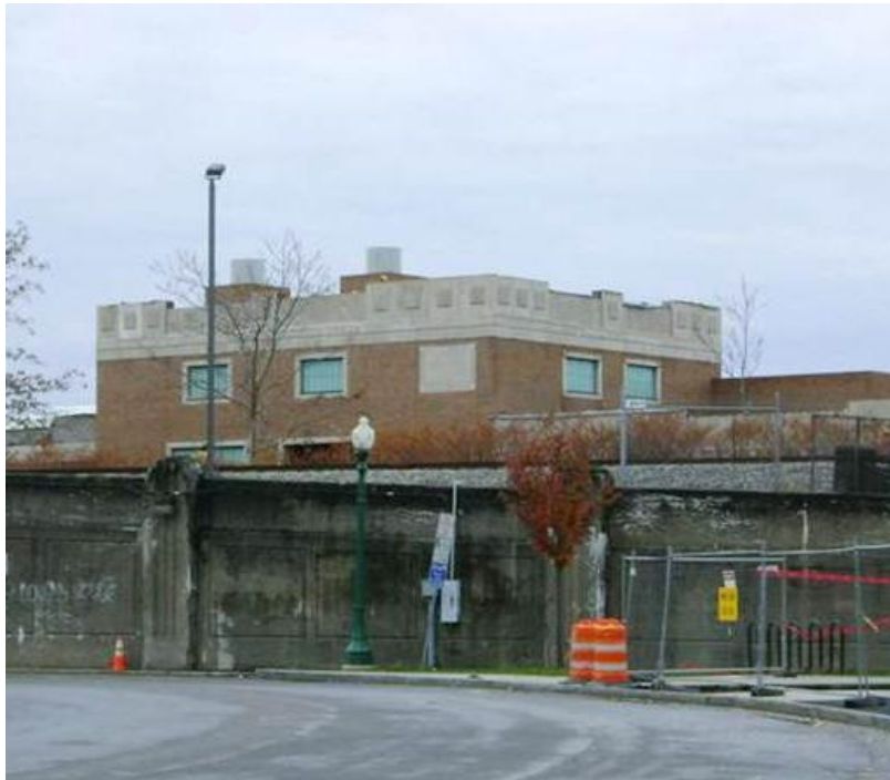
View of Clinton CSO Storage Facility West Chamber from West Jefferson Street November 2013
