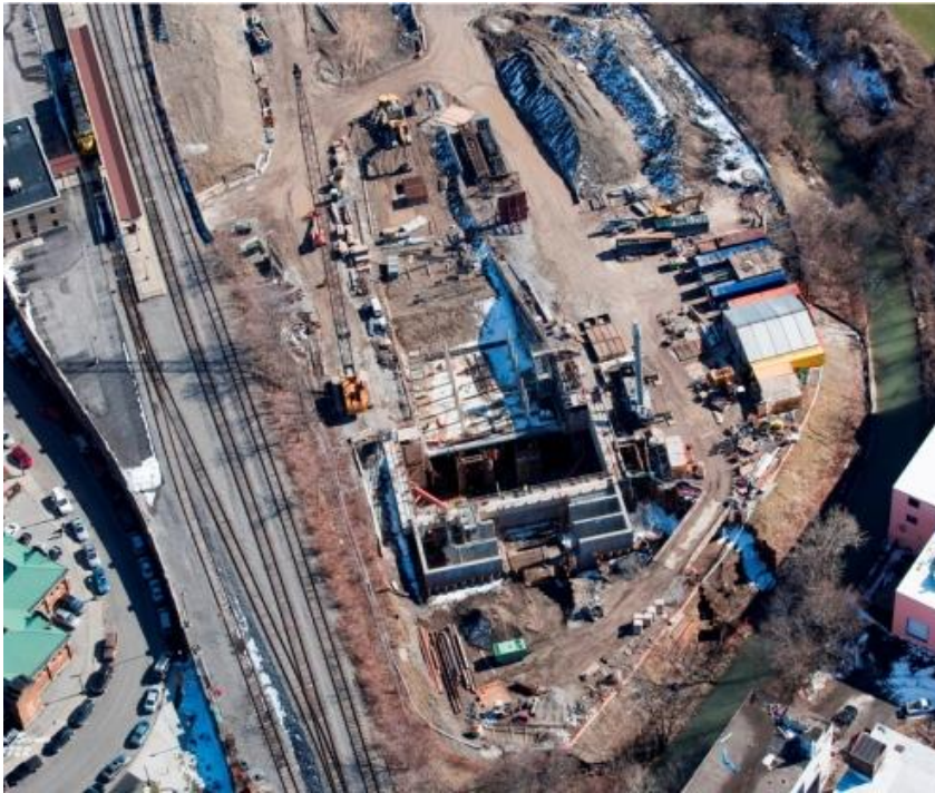
Underground Storage Tank - Concrete Base under Construction (5 Stories below Surface)
