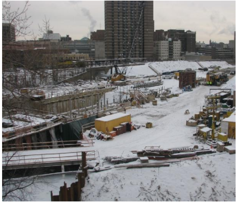
Clinton CSO Storage Facility – Construction 1/25/12
