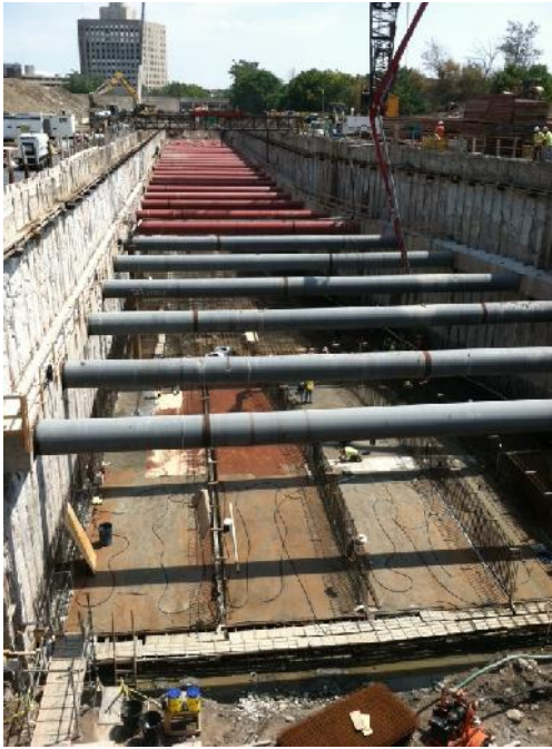
Underground Storage Concrete Base under Construction (5 Stories below Surface)
