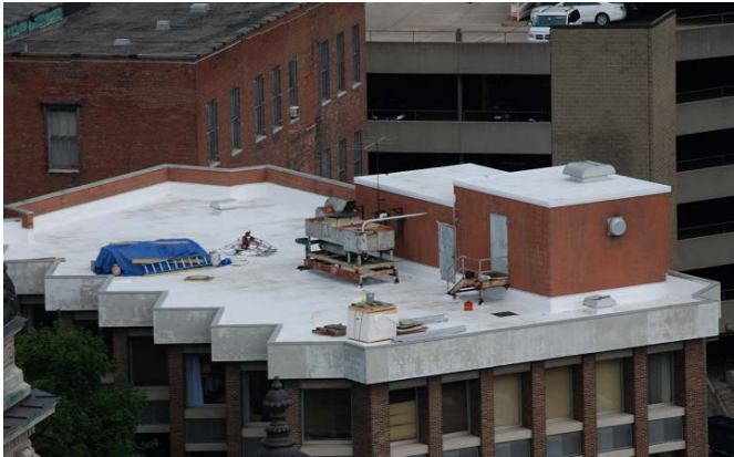
Monroe Building roof before the installation of the green roof
