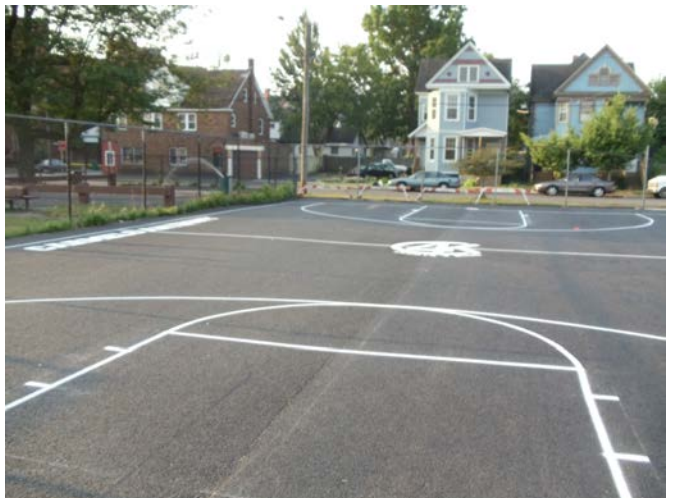
Skiddy Park's new porous pavement basketball courts after the renovation
