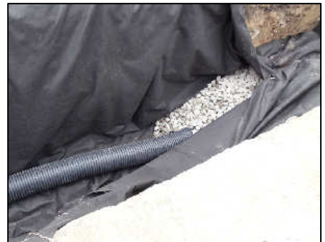
Construction of the underground infiltration trench
