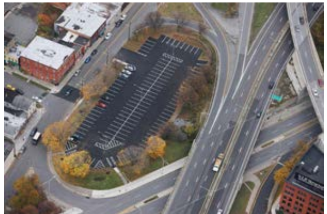
Pearl Street Parking Lot after the renovation & implementation of green
