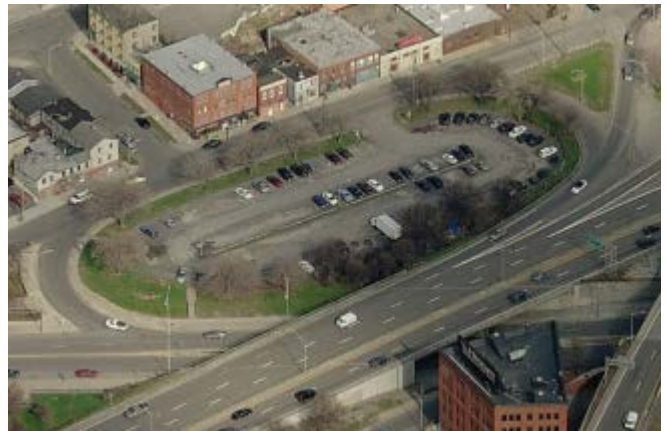
Pearl Street Parking Lot before the renovation & implementation of green infrastructure
