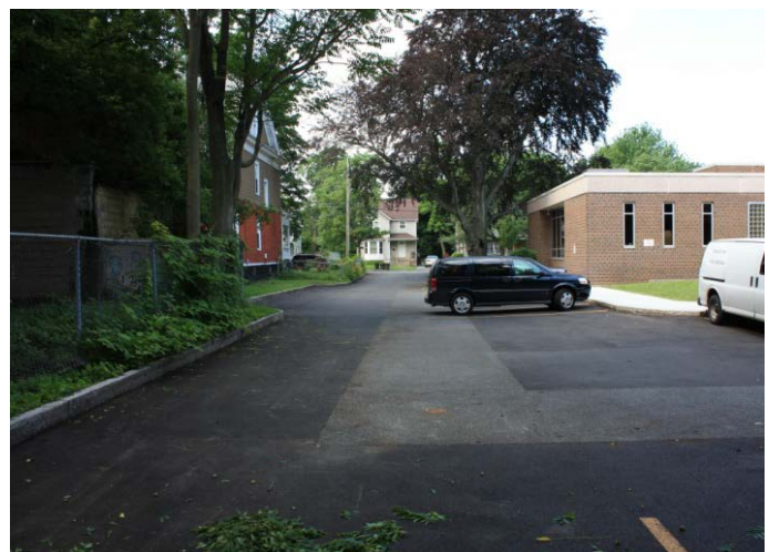
Porous Strip - Parking Lot Entrance
