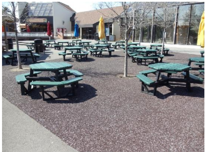
Flexible Porous Pavement in Courtyard
