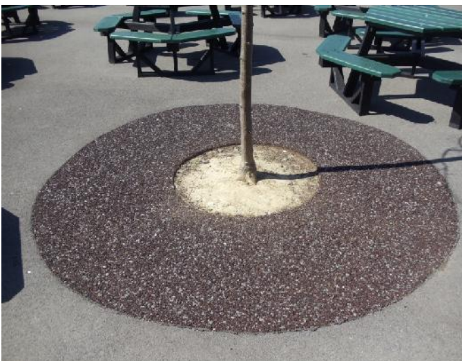
Flexible Porous Pavement Installed Around Trees in Courtyard
