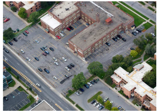
Aerial View of SCSD Central Offices Parking Lot Prior to Construction
