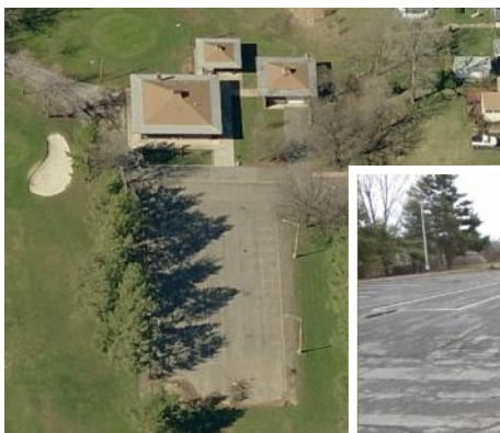
Sunnycrest Golf Parking Lot conditions prior to construction
