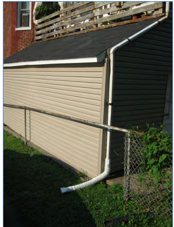
Residential downspout disconnection in Lancaster, PA
