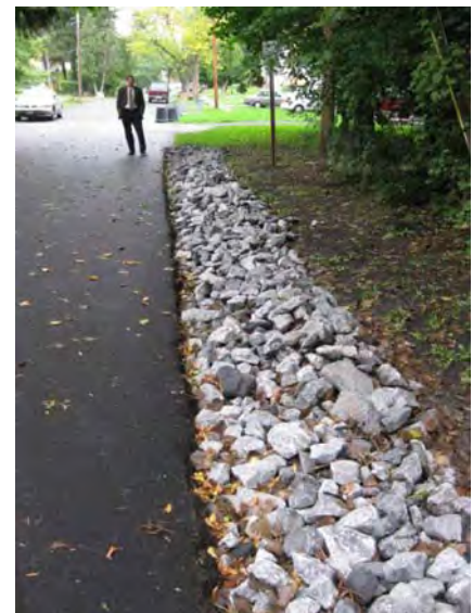
Infiltration trench retrofit at Gorland Ave in Syracuse, NY
