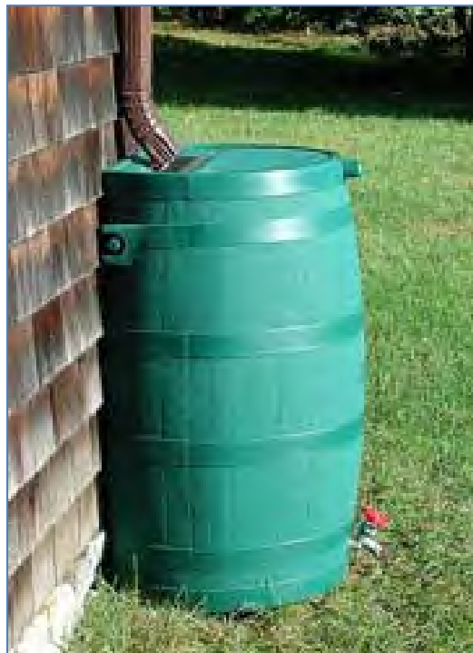
Figure 6: Example of downspout disconnection to rain barrel (Source: Onondaga County, New York <ongov.net>)
