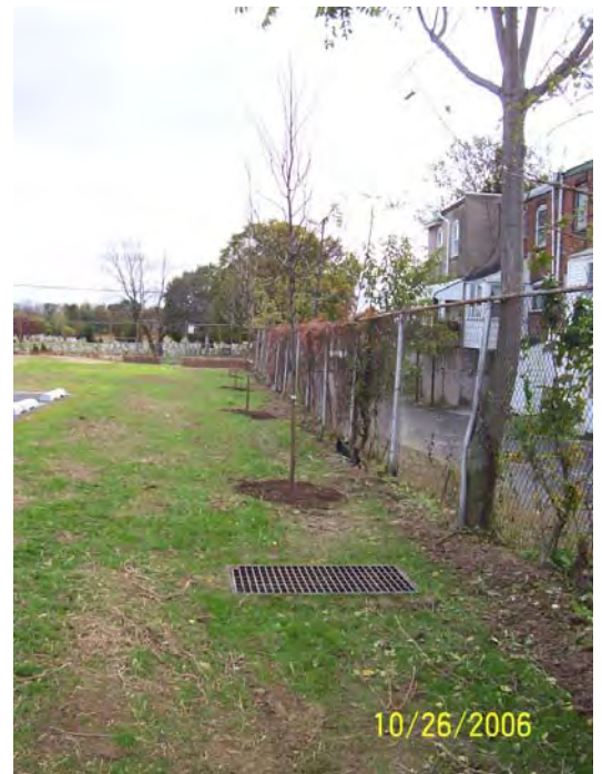
Tree trench located at Upper Darby Park outside of Philadelphia, PA
