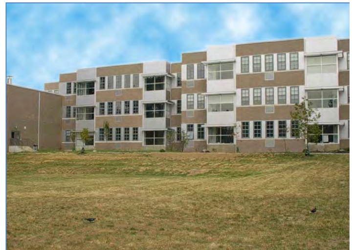
The Subsurface Infiltration Bed beneath this playfield manages rooftop runoff from the adjacent school building, Philadelphia, PA
