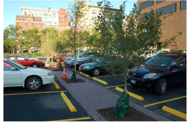
Tree trench with porous pavers and subsurface infiltration bed, located in City Lot No. 21, Syracuse, NY
