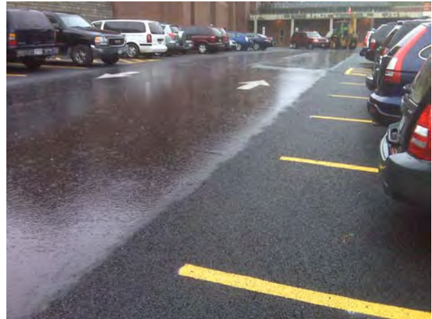
Porous asphalt parking spaces at SUNY ESF parking lot in Syracuse, NY
