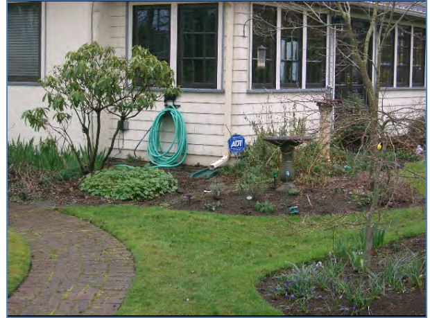
Residential downspout disconnect in Portland Oregon (Source: Portland Stormwater Website)
