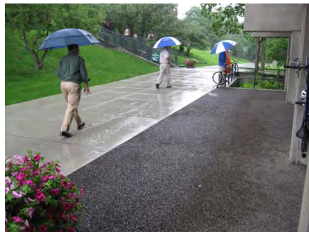
Flexipave installation at SUNY ESF in Syracuse, NY
