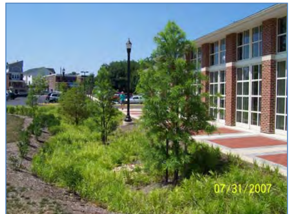
Rain garden at Woodlawn Library in Wilmington, DE.
