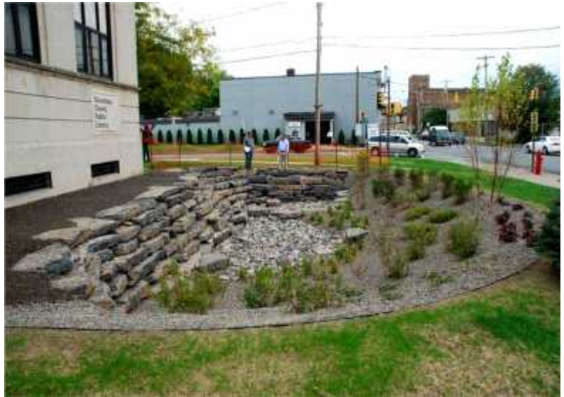
Completed Bioretention Area at Beauchamp Library
