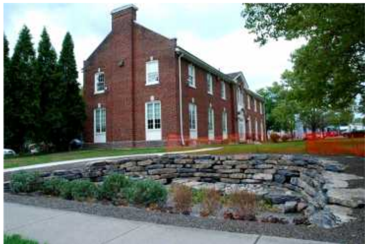
Completed Rain Garden at White Library
