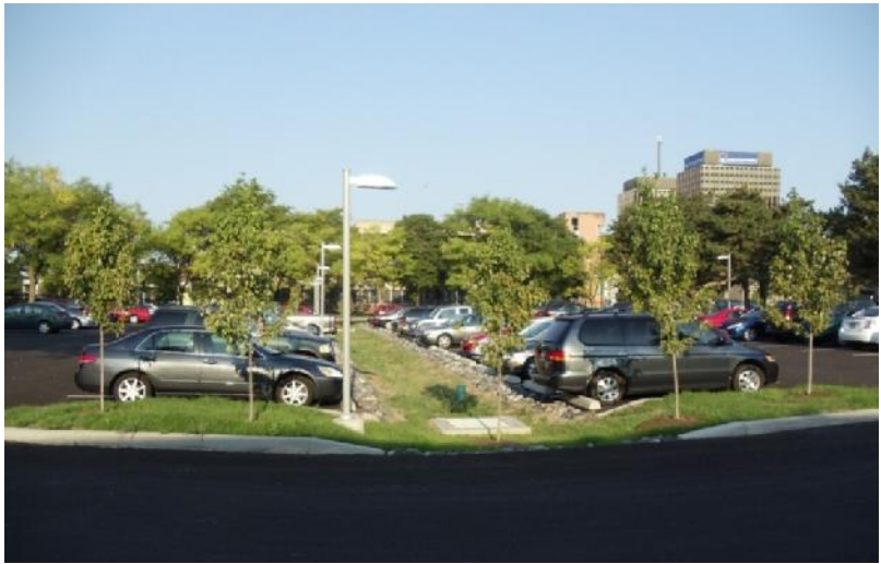
New Parking Lot Median with Vegetated Swale
