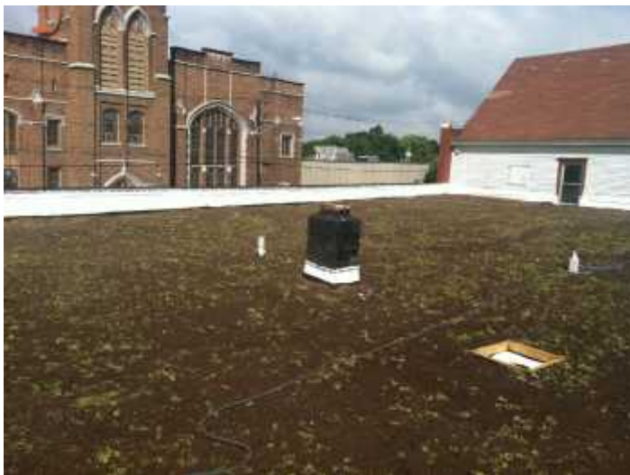
View of Green Roof (Northern view)
