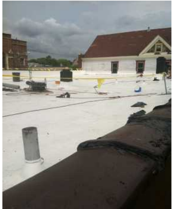
View of Roof before Construction
