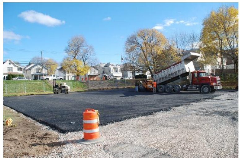
Porous Asphalt Installation for the Basketball Court
