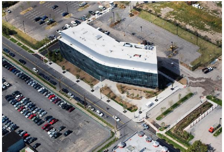
Aerial View of SUNY Upstate Biotechnology Center after Project Completion
