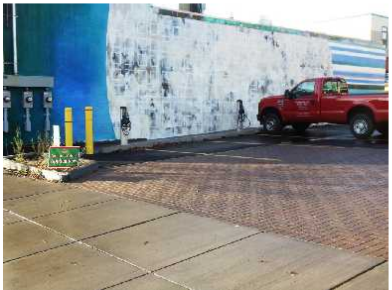
View of Porous Pavers in Parking Lot
