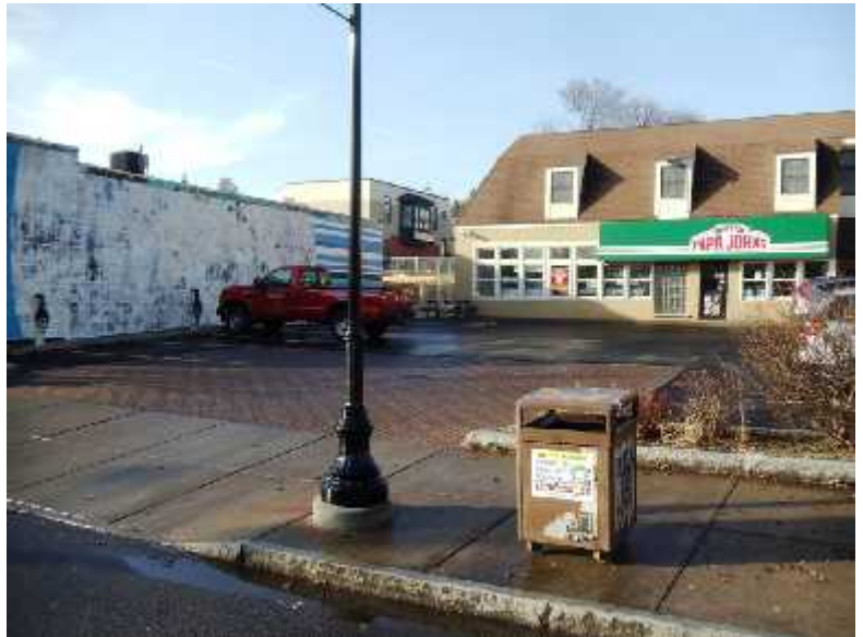
Parking Lot Reconstruction
