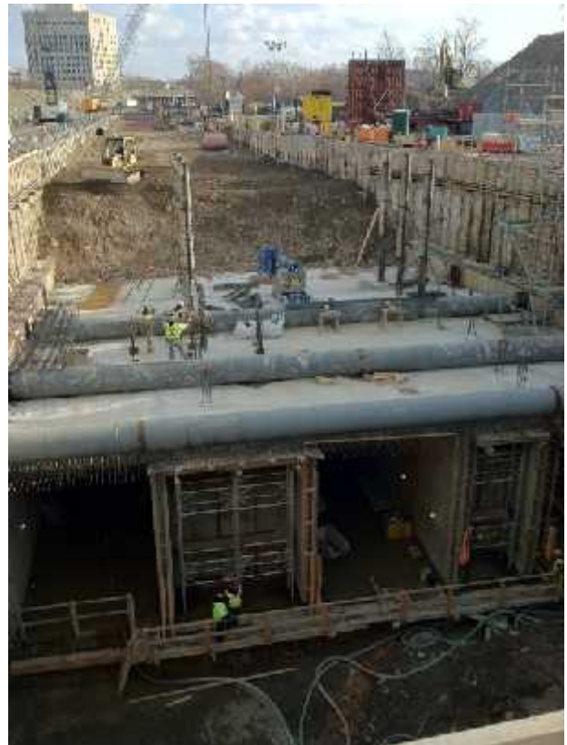
Clinton CSO Storage Facility Construction Backfilling over the Tunnels (12/01/12)
