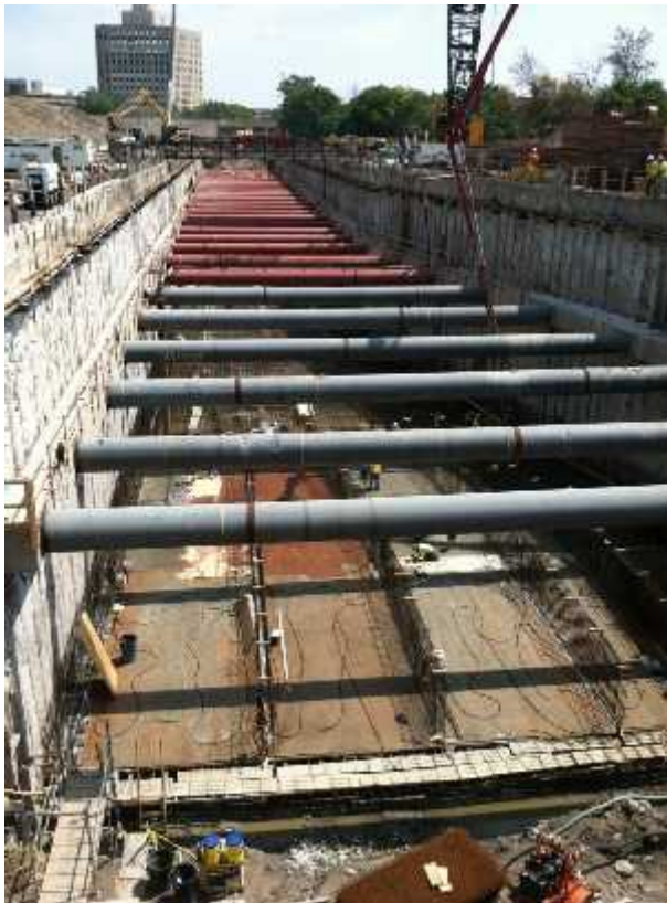
Underground Storage Tank - Concrete Base under Construction (5 Stories below Surface)
