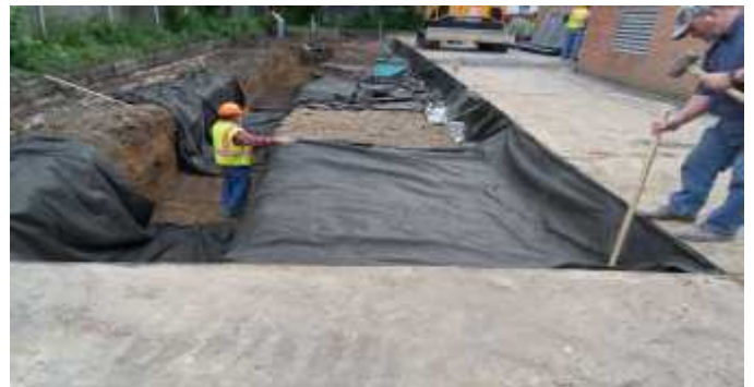
Construction of Infiltration Bed
