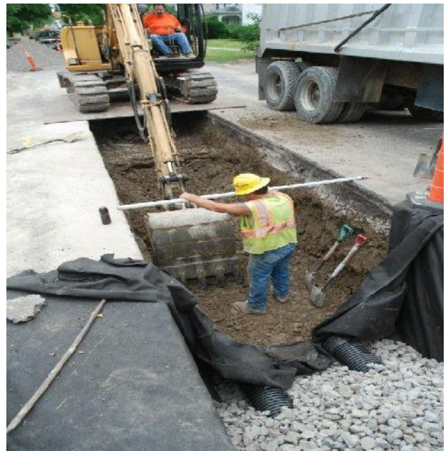
Construction of the Underground Infiltration Trench in the Sumner Ave Road Reconstruction Project
