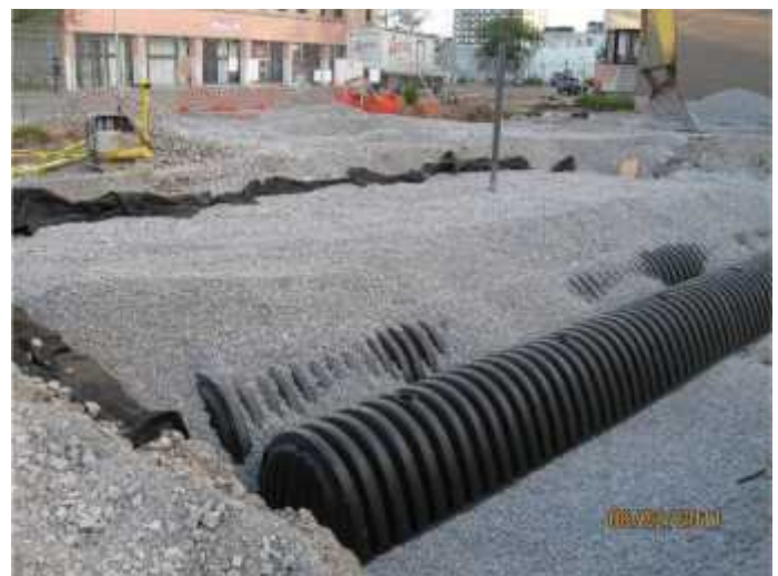
Stone Back-Fill of Chambers Units
