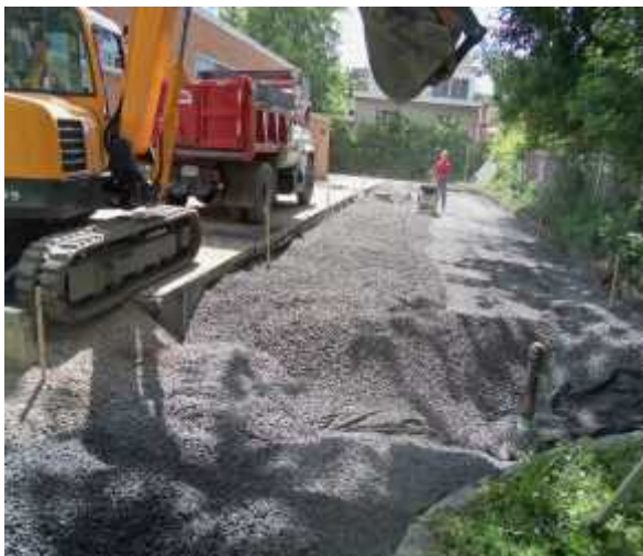
Construction of Infiltration Bed Beneath Porous Concrete
