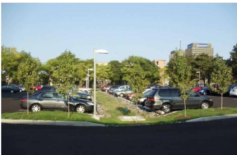
New Parking Lot Median with Vegetated Swale
