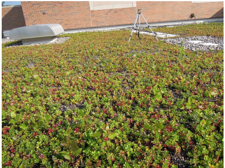
Green Roof at the Clinton Storage Facility
