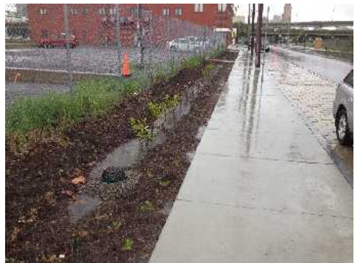
Interlocking Porous Paver Parking Lane and Bioswale on Southern Side of E. Washington St.
