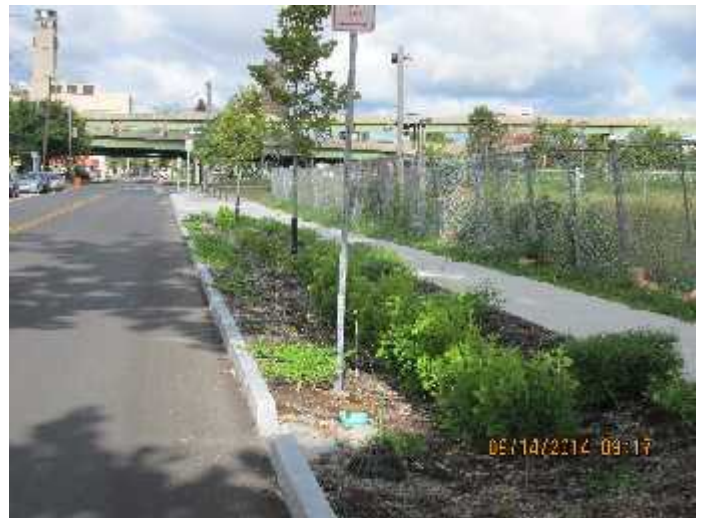
Completed Bioswale on the North Side of E. Washington St.
