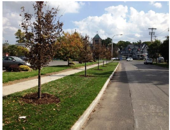
Bioswale Installed on Slocum Avenue
