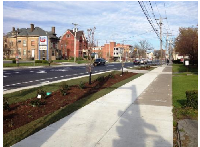
Completed Photograph of West Onondaga Street
