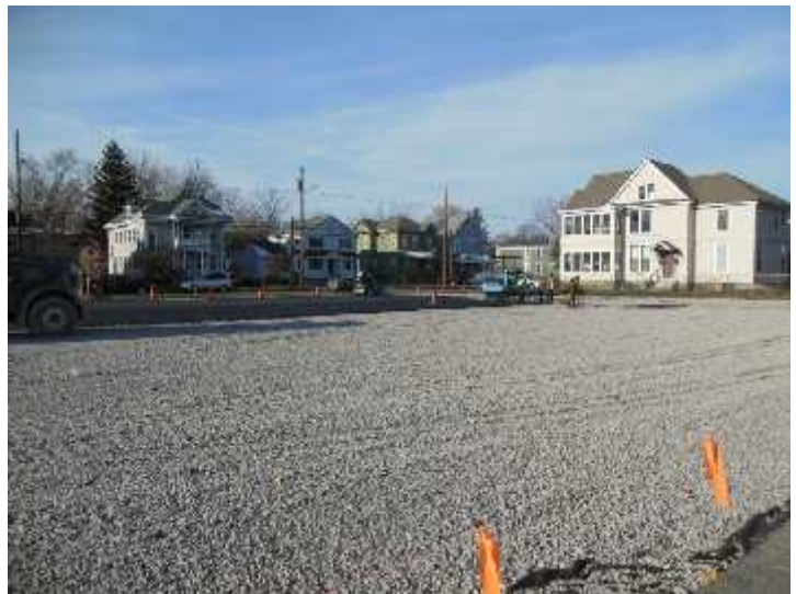
Installation of Subsurface Drainage Material and Porous Sub-Base
