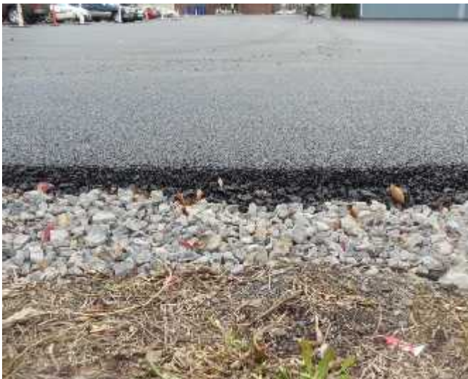
Cross Section of Porous Pavement
