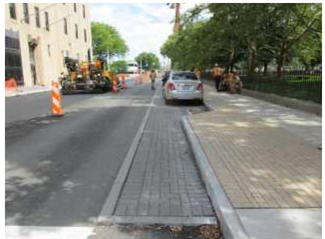
Porous Paver Parking Lane and Snow Storage Area on E. Genesee St at Firefighters Memorial Park
