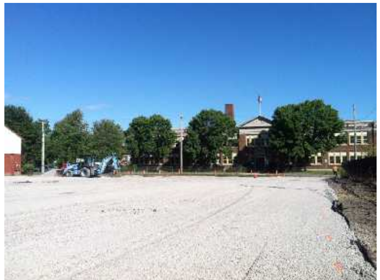
Installation of Subsurface Drainage Material
