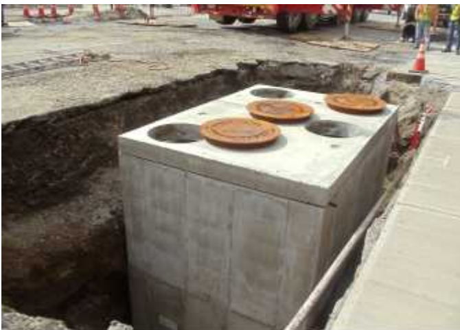
Manufactured Treatment Device Installed in the Spring of 2014
