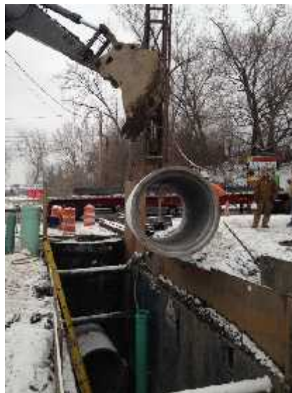
Installation of the 48-inch reinforced concrete pipe on a pipe cradle upstream of manhole HW-6.
