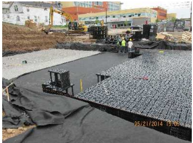
Installation of Underground Infiltration System
