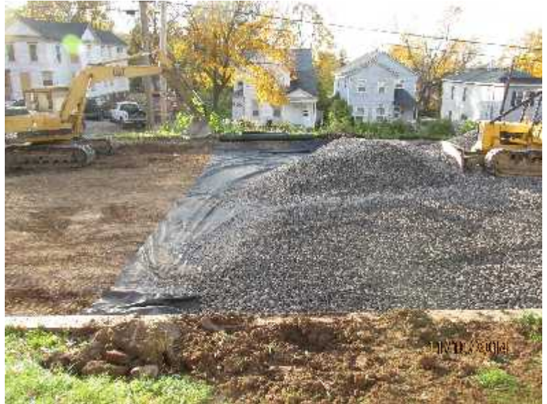
Installation of Underground Infiltration System
