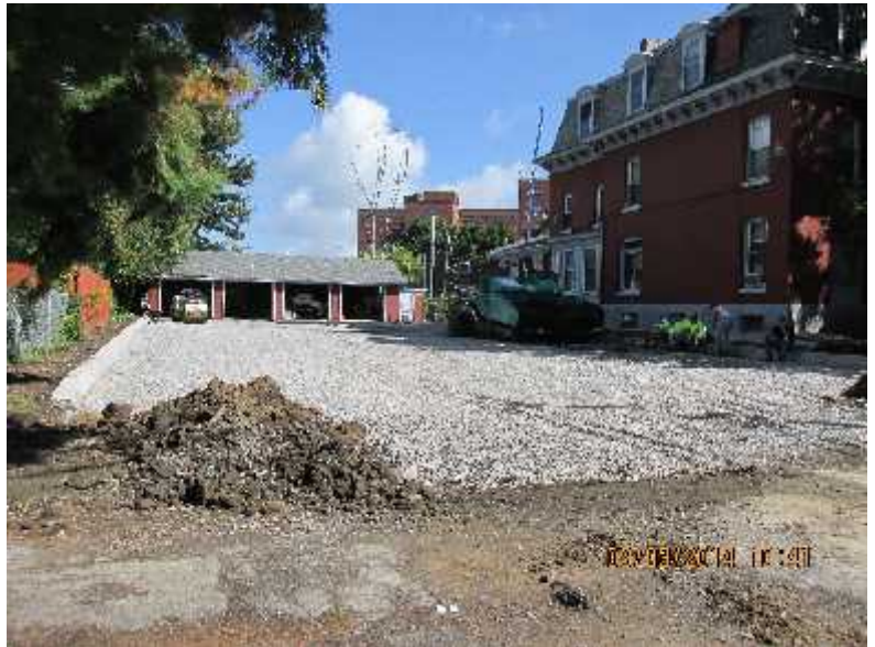
Porous Pavement Parking Lot during Construction
