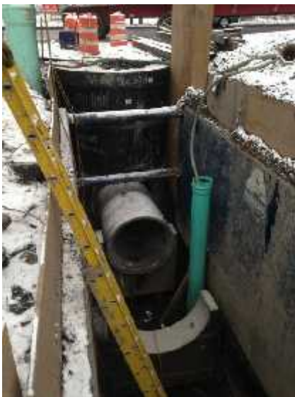
Installation of the 48-inch reinforced concrete pipe on a pipe cradle upstream of manhole HW-6.
