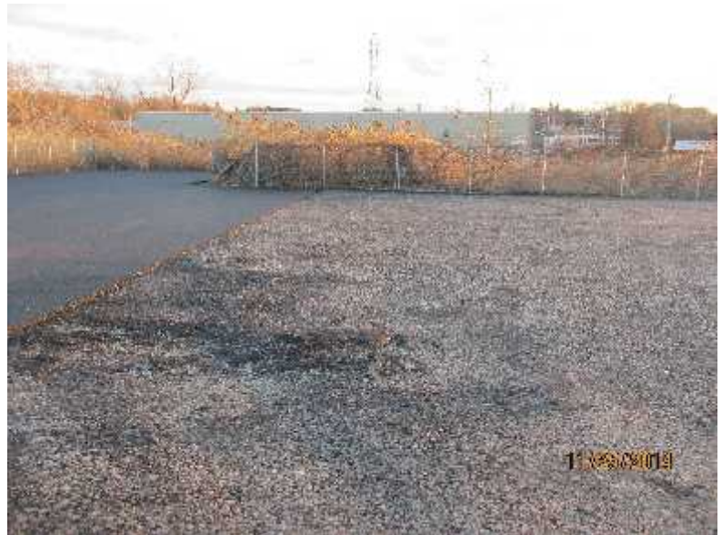
Installation of Drainage Material
