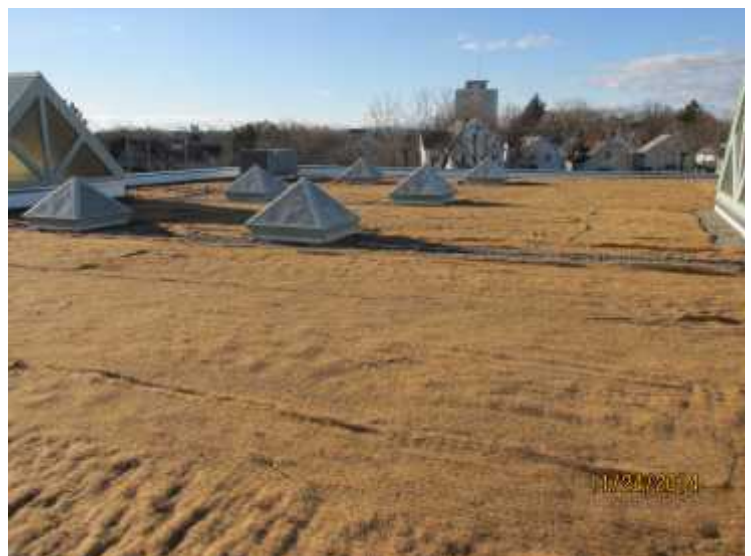
Upper Green Roof Upon Completion; Wind Blanket Installed to Protect Sedum Cuttings
