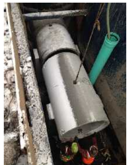
Installation of the 48-inch reinforced concrete pipe on a pipe cradle upstream of manhole HW-6.
