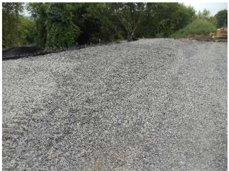
Subsurface Drainage Material for Porous Asphalt
