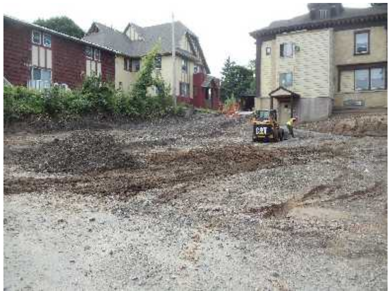
Construction of Porous Pavement Parking Area
