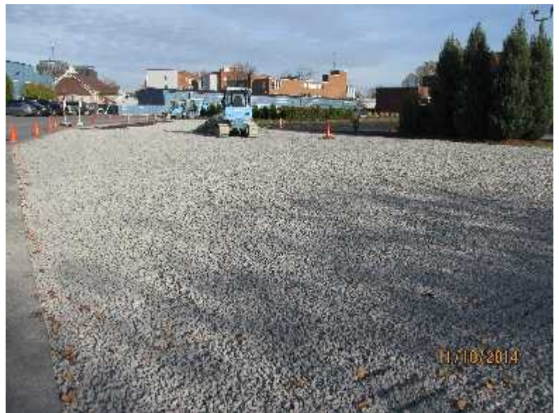
Installation of Subsurface Drainage Material
