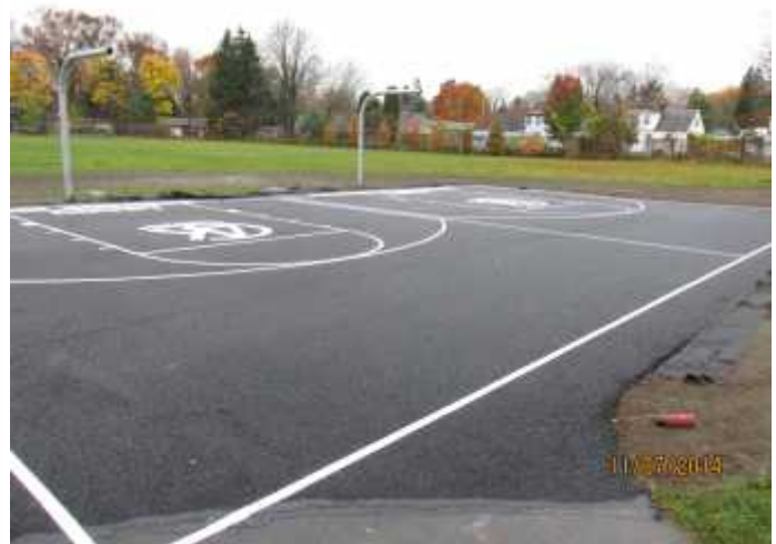
Completed Porous Asphalt Basketball Court
