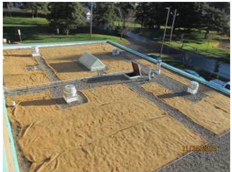
Lower Green Roof Upon Completion; Wind Blanket Installed to Protect Sedum Cuttings
