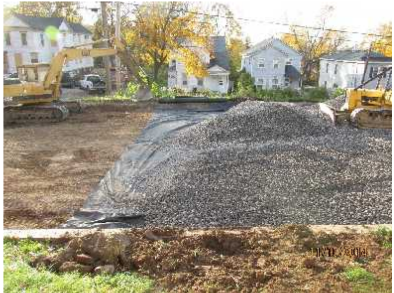
Installation of Underground Infiltration System
