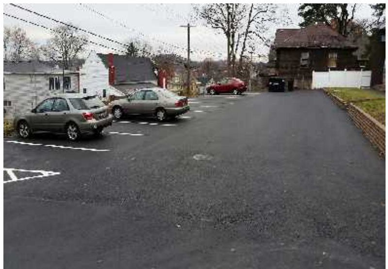
Porous Pavement Parking Area
