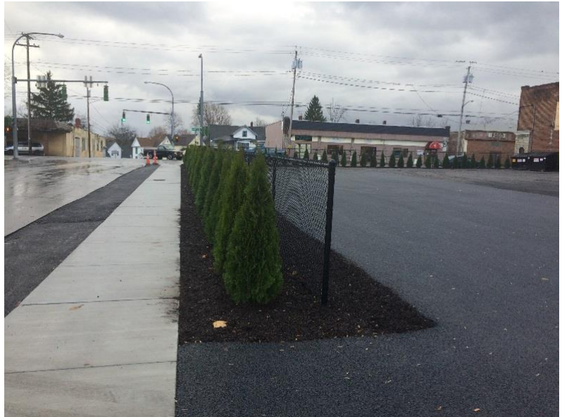
Pavement Removal and Porous Asphalt Surrounding the Parking Area
