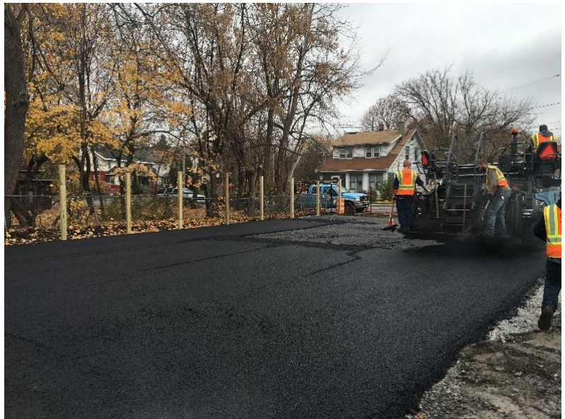
Porous Asphalt Installation
