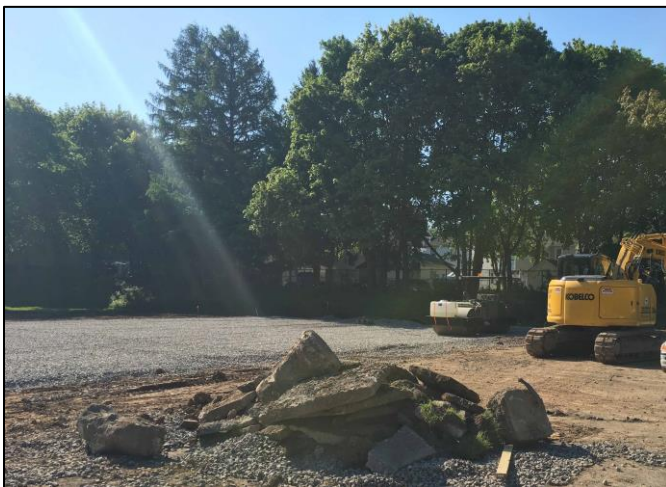
Porous pavement basketball court construction
