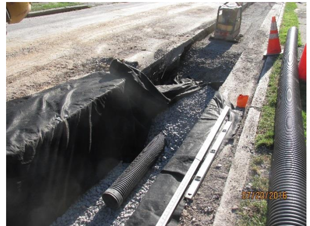
Typical Underground Infiltration Trench Construction (West Colvin Street, 2016)
