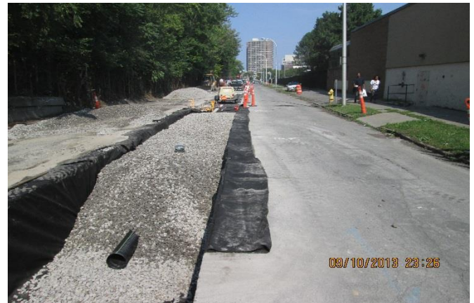
Typical Underground Infiltration Trench Construction (Clinton St., 2013)
