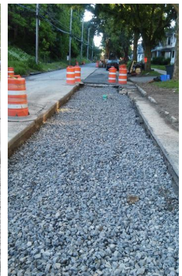
Lancaster Ave Infiltration Trenches
