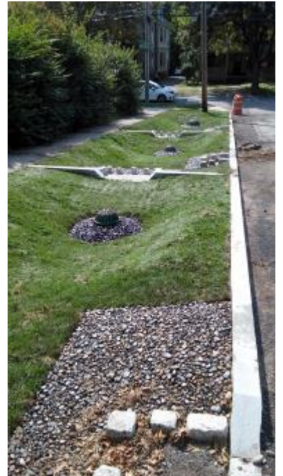
Lancaster Avenue Vegetated Infiltration Swale
