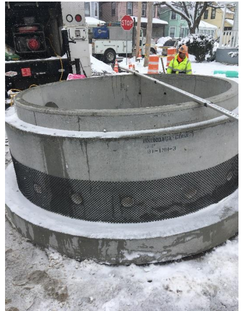
Infiltration Manhole Before Installation
