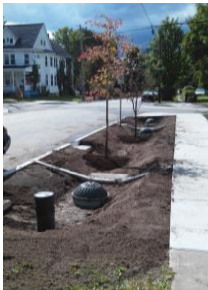
Ackerman Avenue Vegetated Infiltration Swale
