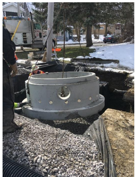
Infiltration Manhole Before Installation
