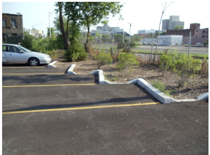
Bio-retention area - parking lot view
