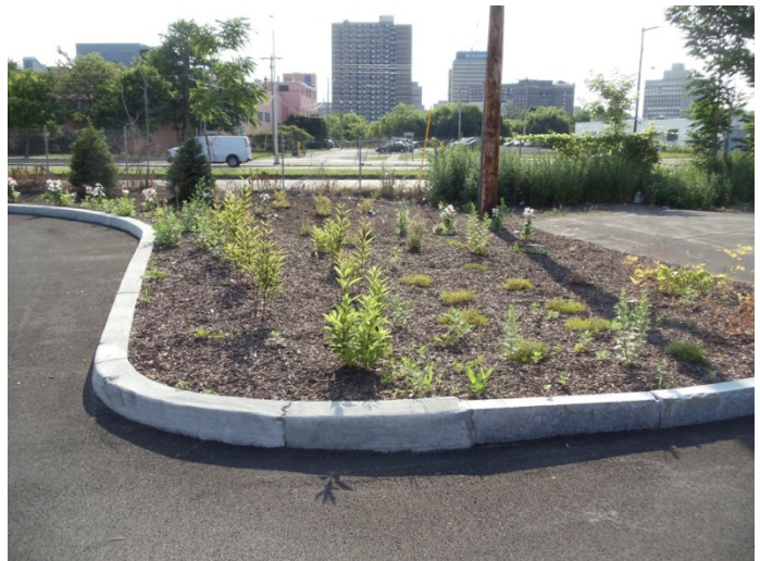
Bio-retention parking lot facing east
