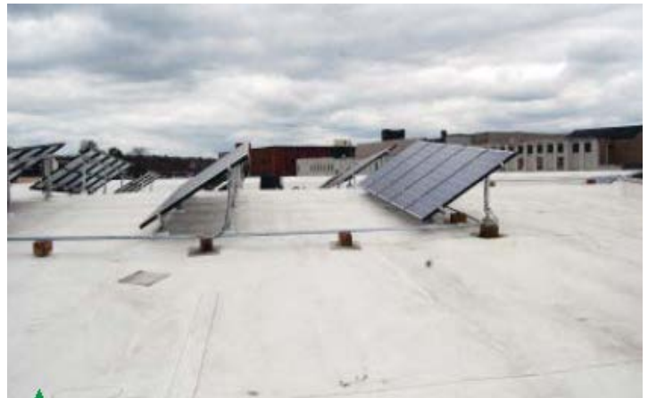
View of roof top before (solar panels are part of a separate project)
