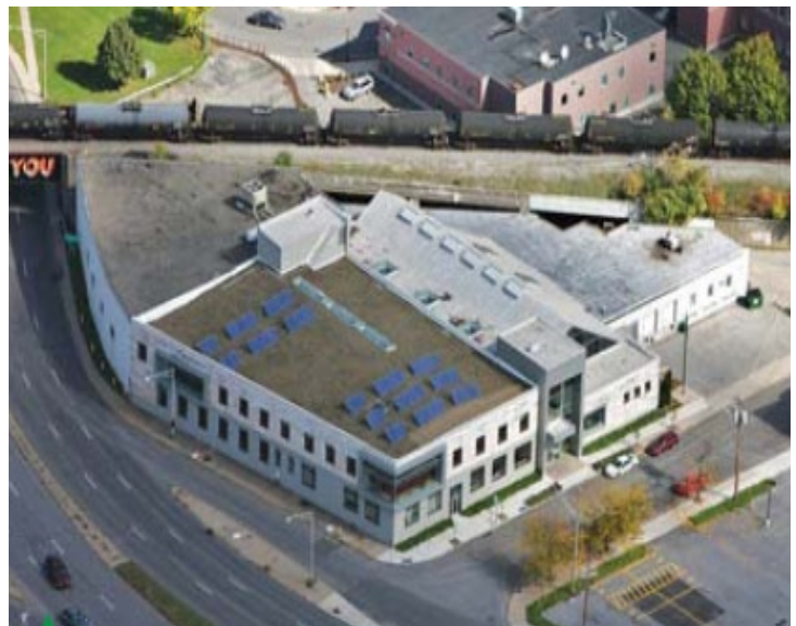
Rooftop with green roof installed
