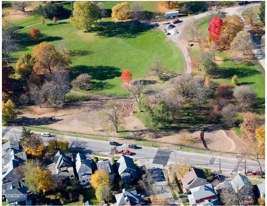
Avery Ave Rain Gardens under Construction
