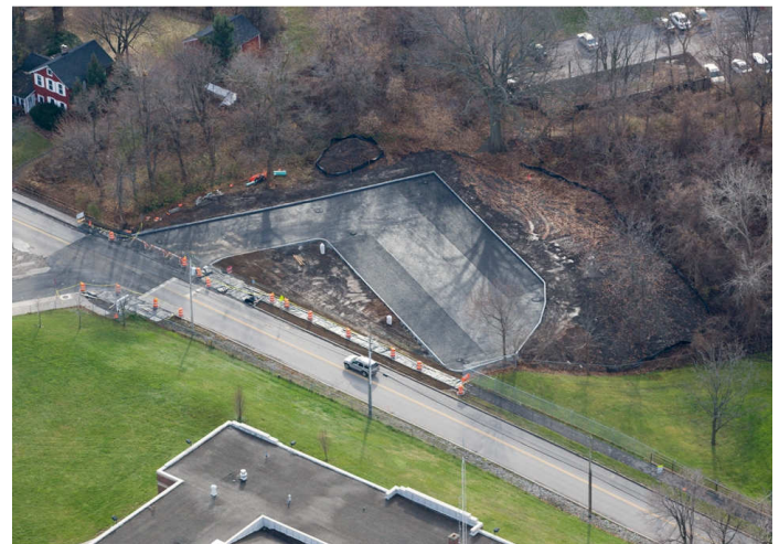
Porous Lot - Construction Nearing Completion
