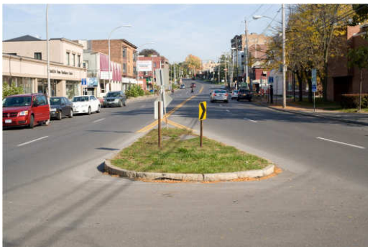
E Genesee St Before Construction
