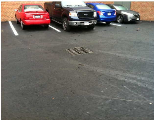
View of Infiltration Catch Basin
