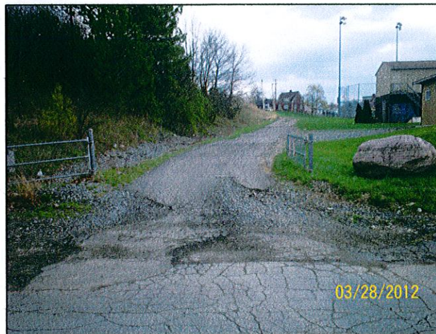
PARK ACCESS ROAD
