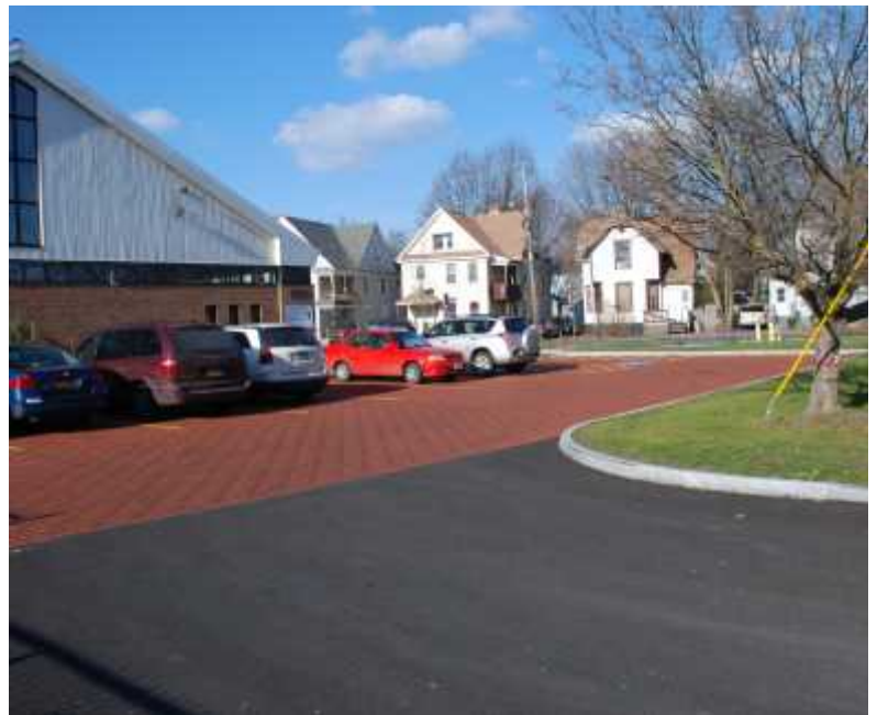
Porous Pavers in Mundy Library Parking Lot
