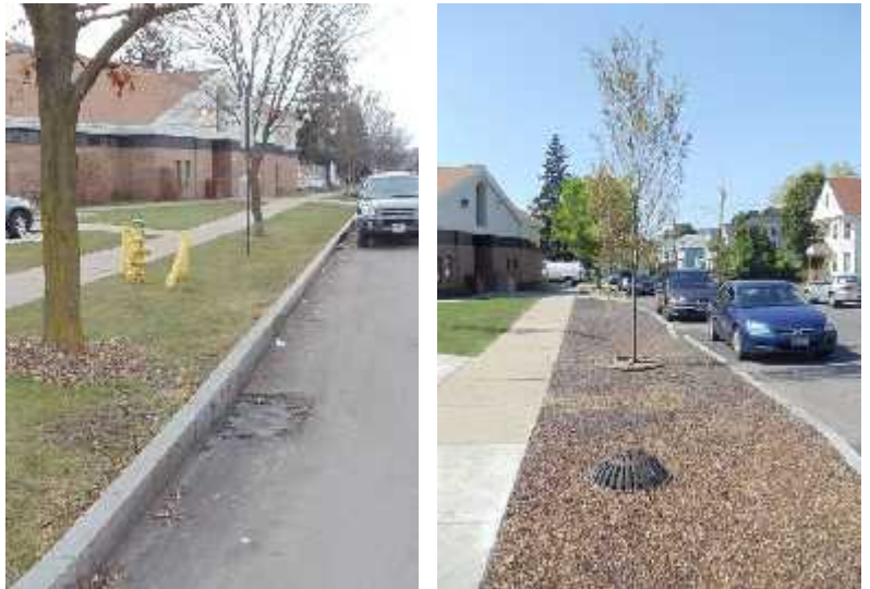
Before and After Construction Photos of Tree Trench along Rowland Street
