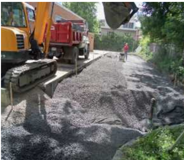
Construction of Infiltration Bed Beneath Porous Concrete
