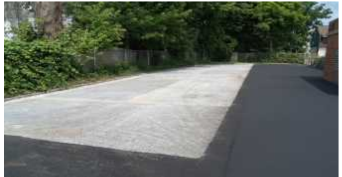
Porous Concrete Area Behind Petit Library
