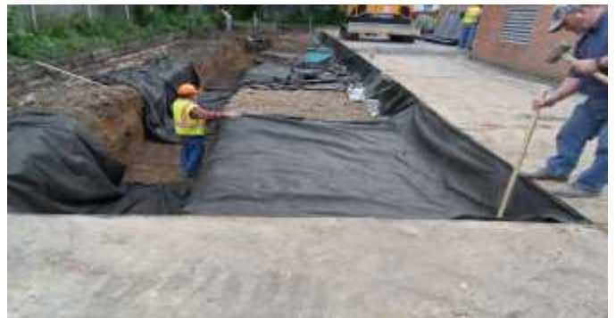
Construction of Infiltration Bed
