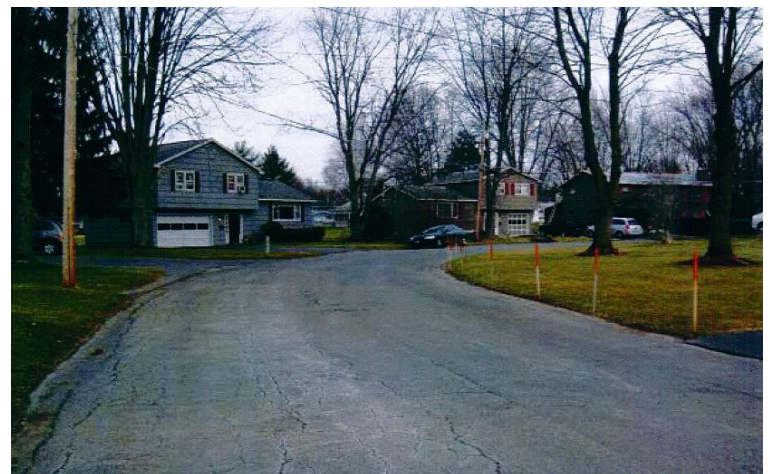
Hummingbird Path Road Conditions before SGIP Project Implementation
