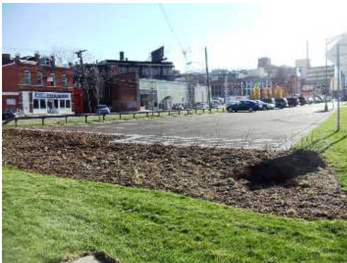
Porous Pavement and New Bioretention Area at Northern End of Lot 4
