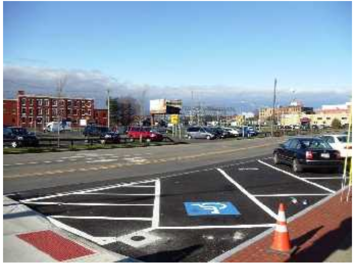
New Porous Pavement Parking Lane across from City Lot 4
