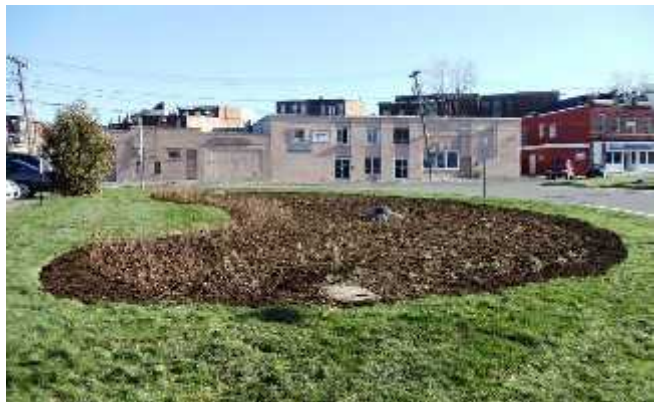
Bioretention Area on NYSDOT Property
