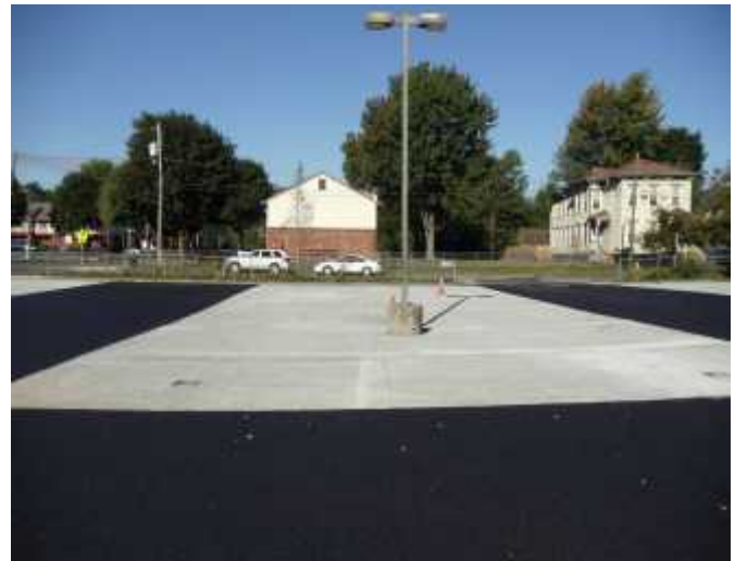
Parking Lot after Construction
