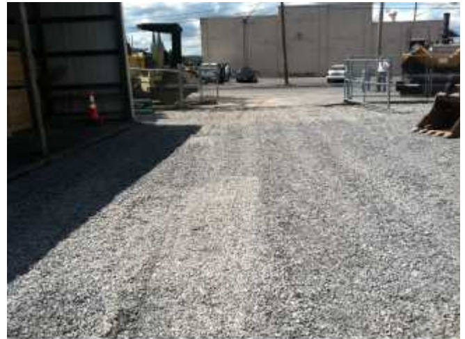
Parking Lot During Construction
