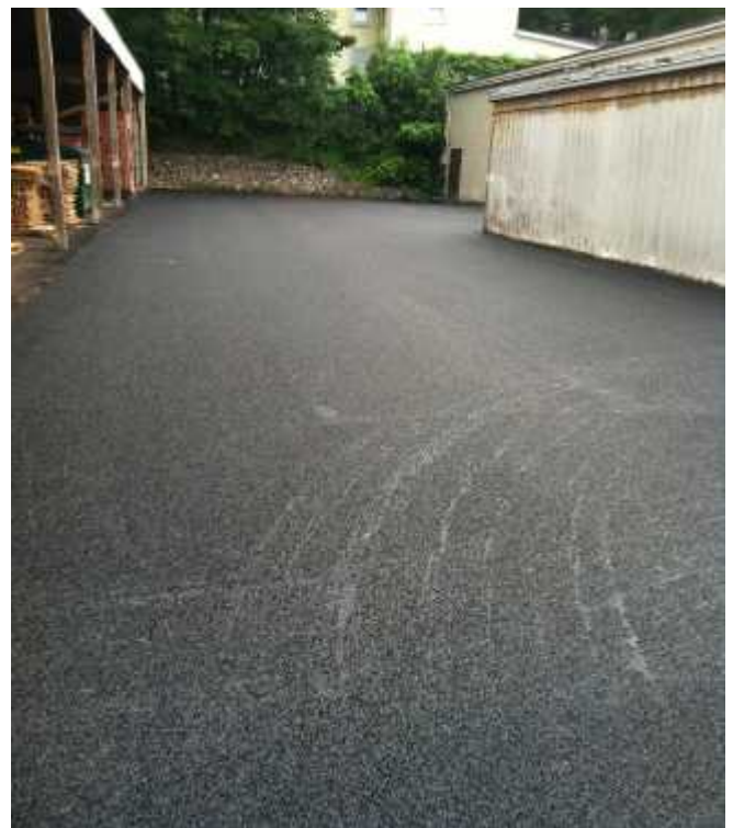
Parking Lot Project Completed
