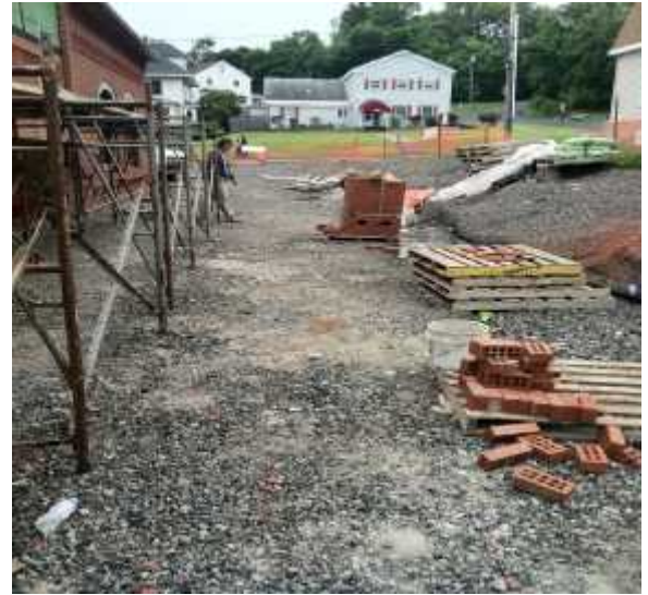
The East Side of the Building During Project Construction
