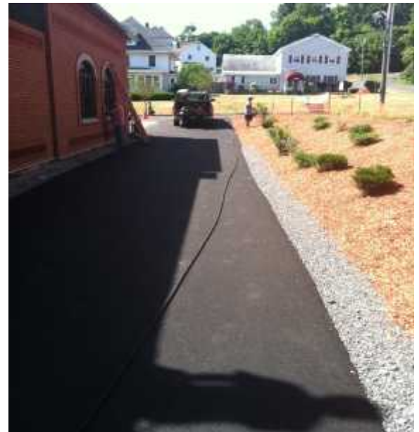
The East Side of the Building after Project Completion
