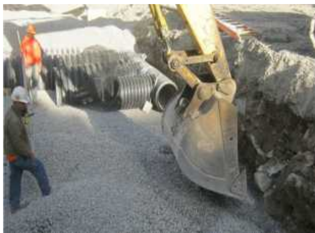
Excavation of Underground Storage
