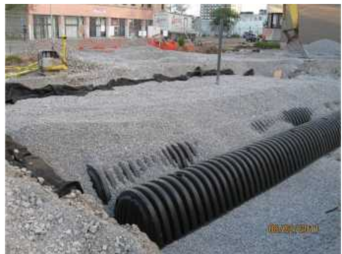
Stone Back-Fill of Chambers Units
