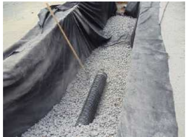
Construction Photographs of the S. State Street underground infiltration trench
