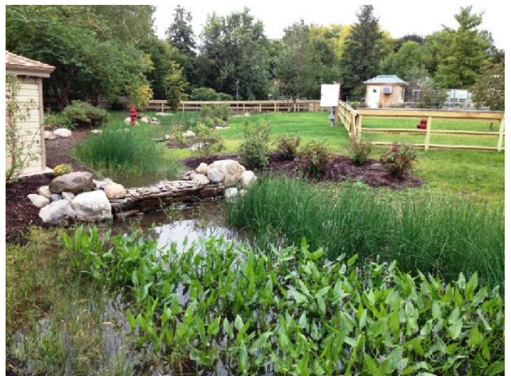
Stormwater Wetland with flow entering from Open Stream Channel
