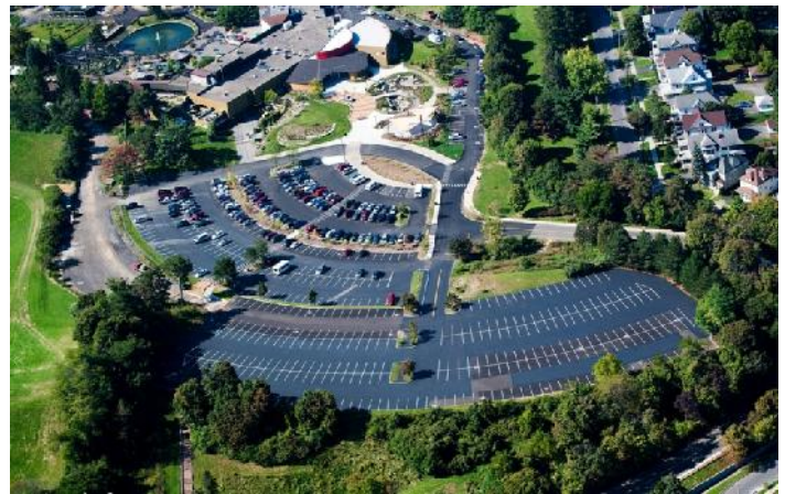
Aerial Photograph of the Rosamond Gifford Zoo Parking Lots nearing Completion
