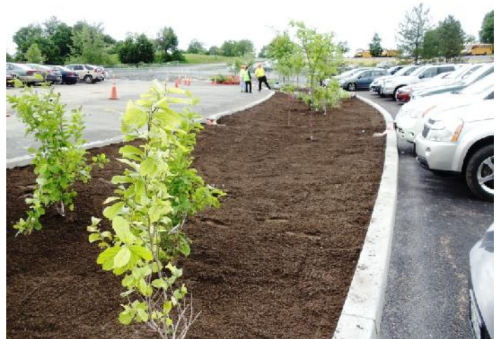
Bioswale and adjacent Porous Asphalt Parking Lane During Construction
