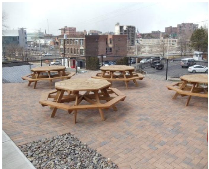
Porous Paver Patio Behind Facility
