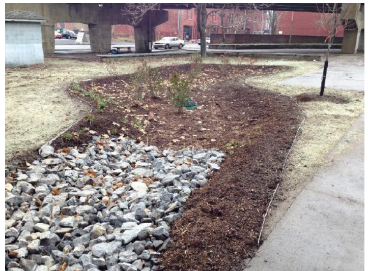
Constructed Bioretention Area at Site 5
