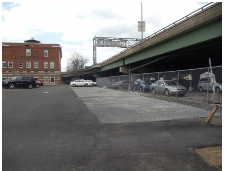
New Porous Concrete Parking Area
